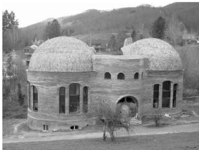
Above: The Glashaus after the renovation
